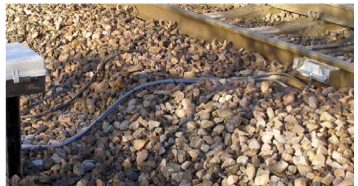
The above image displays assembled parts on site
