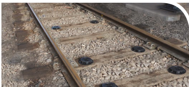
1. Attach pedestals to the sleepers
